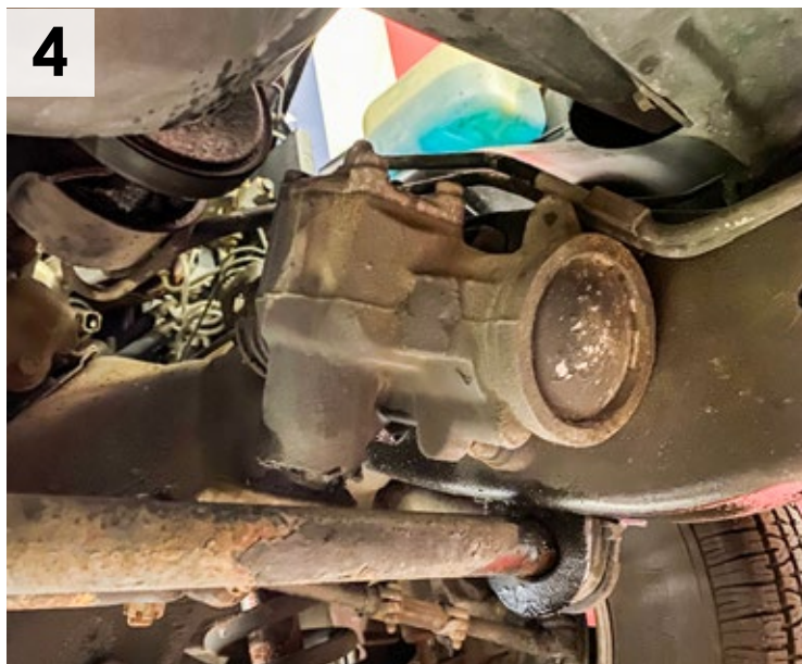
4 Disconnect the pressure and return line from the steering box. Next, remove the bolts that attached the steering box to the frame. Then remove the steering box from the truck.
